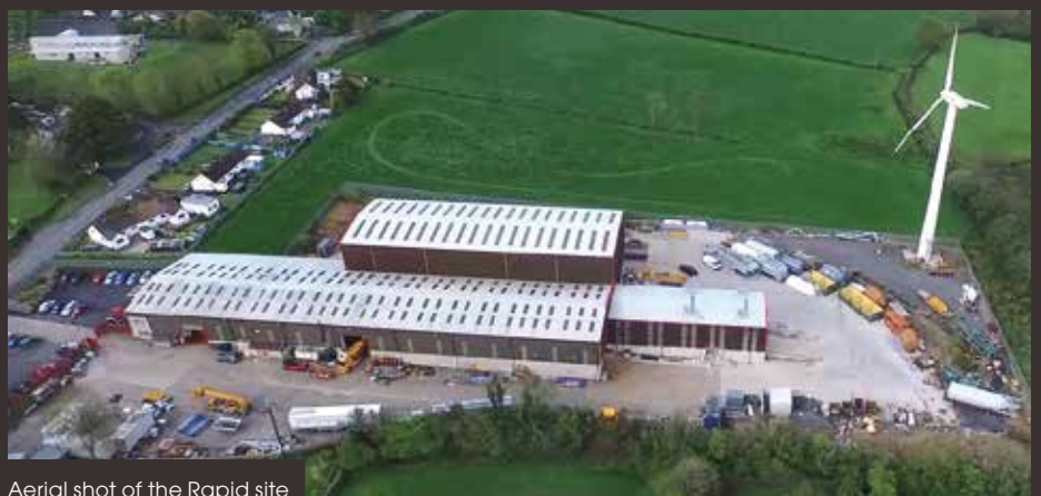
Aerial shot of the Rapid site
