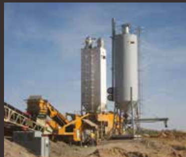
Soil stabilisation California
