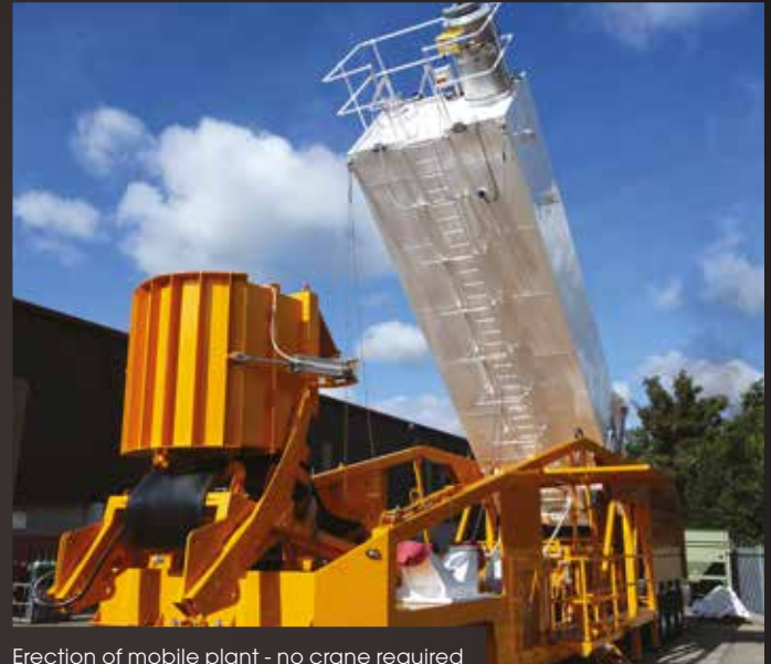
Erection of mobile plant - no crane required
