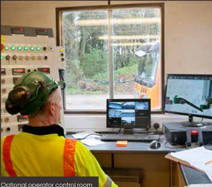
Optional operator control room
