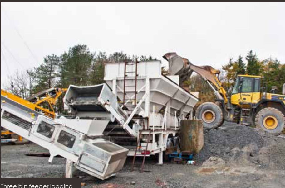
Three bin feeder loading
